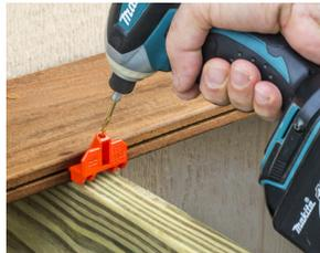
**Step 2:** Predrill using the EB-GUIDE drill guide.
