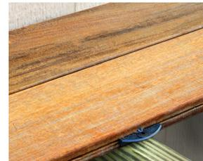
**Repeat Step 2:** Apply construction adhesive to the joint. Slide adjoining deck board onto exposed EB-TY Premium radius sides. Repeat Steps 2 and 3 and install last board using Step 1.
