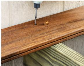
**Step 1:** Install first board by applying construction adhesive and screwing and countersinking directly into the face of the deck board and into the joist; glue an ipê plug in the hole.
