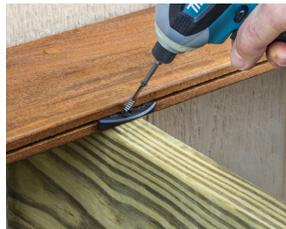
**Step 3:** Place EB-TY Premium™ in deck board groove. Fasten with trim-head screw (included) through the EB-TY and deck board and into the joist.
